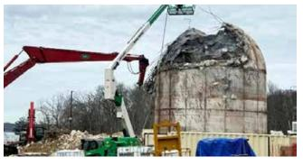
We are decommissioning and dismantling Fort Belvoir's SM-1 Reactor, the first US nuclear reactor to provide sustained power to a commercial electrical grid.
